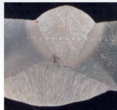
Insufficient penetration and excessive reinforcement; also misaligned.
